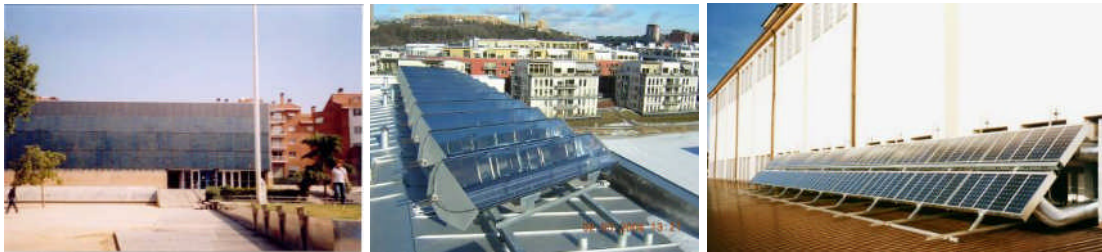
Figure 1: (a) Ventilated PV façade of the Mataro public library in which the heat is recovered and used for space heating and solar cooling, (b) concentrating PV/T system (Vattenfall), (c) PV/T air collector (Grammer KG).
